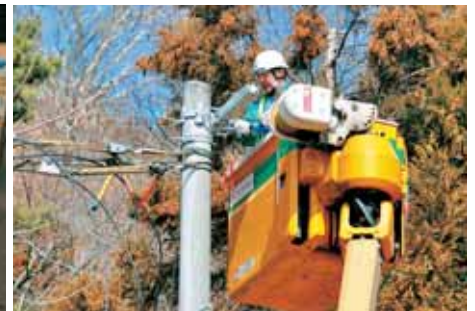
Electricity company sta working on recovering electricity. (Photo: March 19, 2011)
